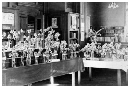
1925 Daffodil Show in the Takoma DC Library.
